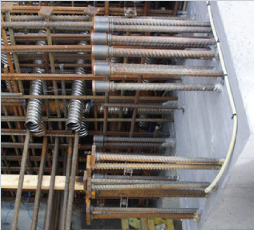
HRC 420 used in construction joint
