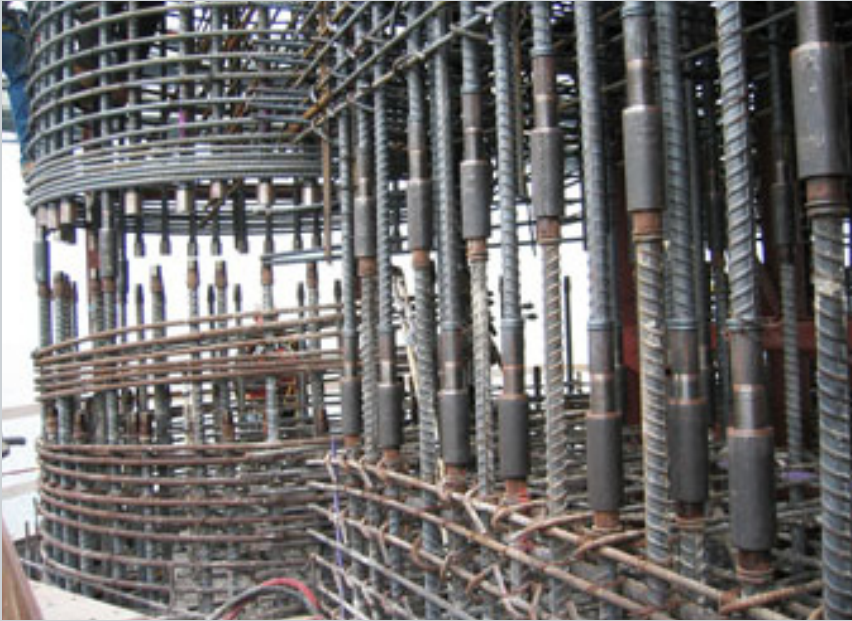
Connection of prefabricated reinforcement units with HRC 400 couplers
